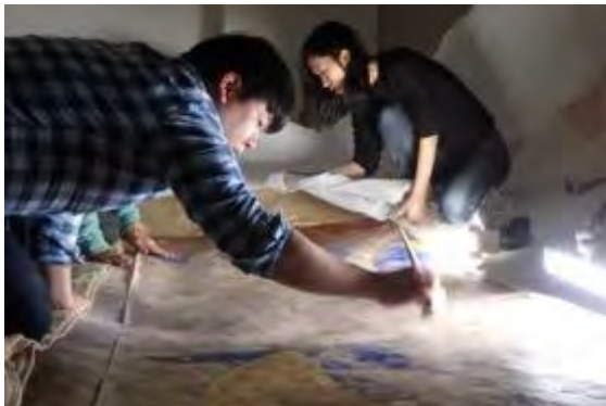
Figure 14: Attaching the printed Japanese washi paper to the structure of the niche
